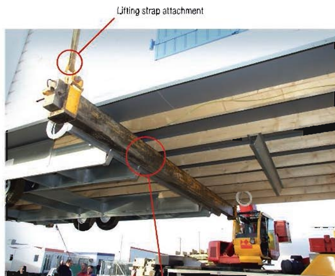
Lifting bar perpendicular to the cross-members and close to the central metal part
